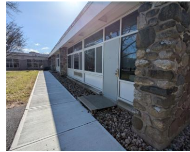
Landing and step at classroom doors to exterior 1960/64 door.
