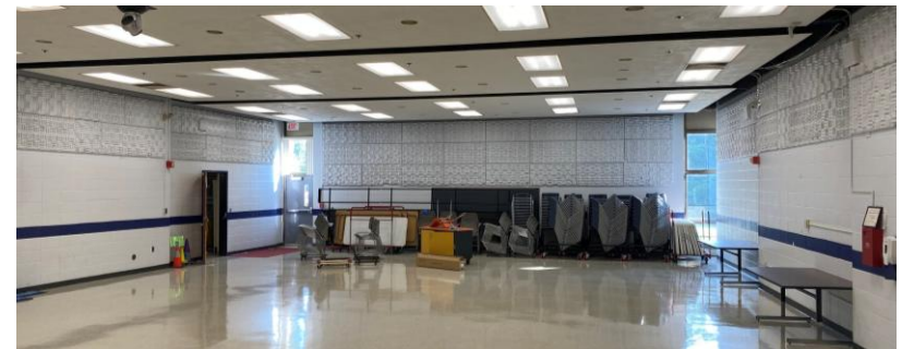
South Assembly walls
