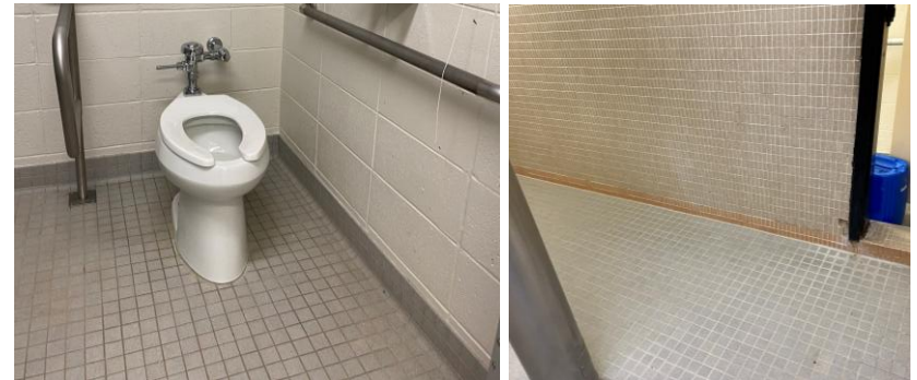
Typical tile flooring at toilet rooms and locker rooms
