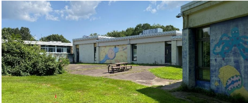
West elevation transition from the 1970 wing to the 1960/196 wing
