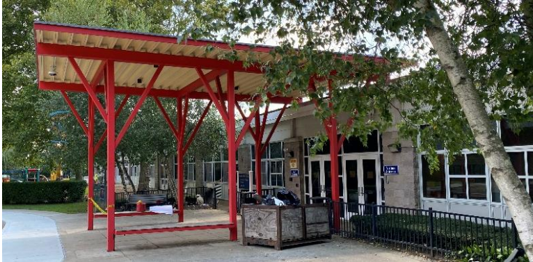
North entrance canopy
