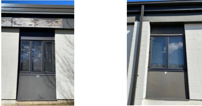
Typical windows at the 1994 addition
