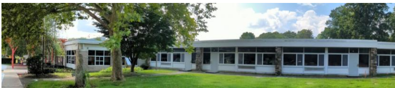
1960 and 1964. Metal panels and river rock façade
