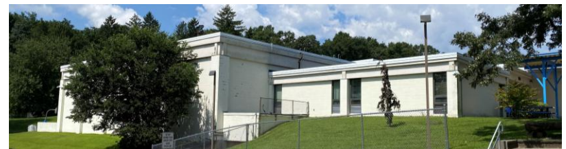
1970. South west façade. Painted CMU.
