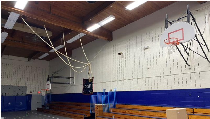
South Gymnasium walls
