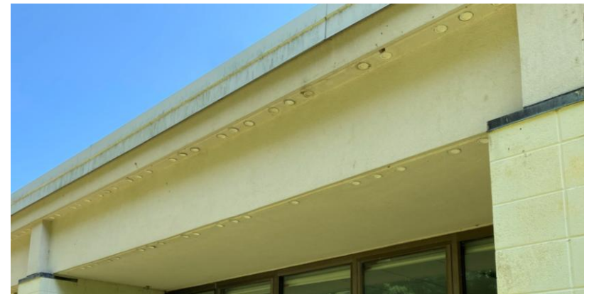
Soffit vents
