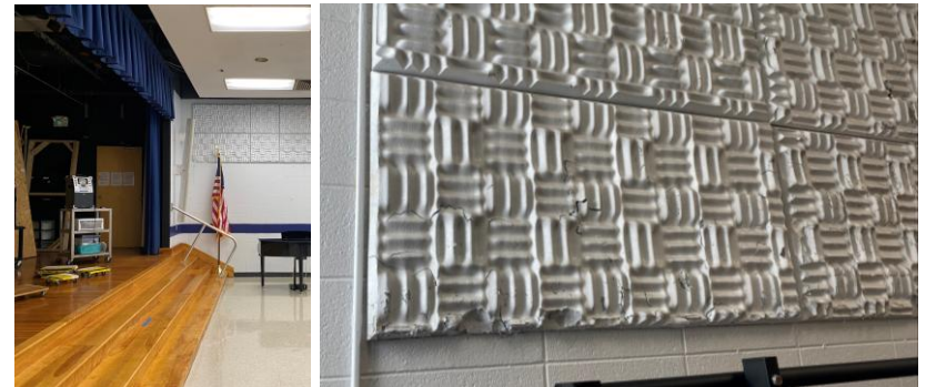
South Assembly stage area Typical acoustic wall panel
