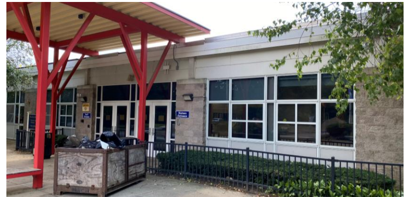
1997. Split face CMU and storefront windows at north entry façade
