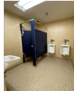
Typical 1970's ganged toilet
