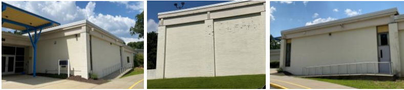
1970. Painted masonry exterior walls.
