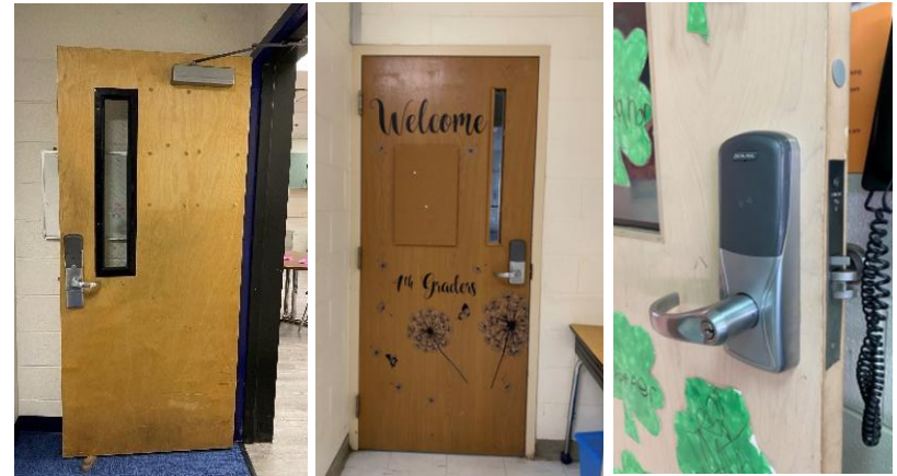
Typical Classroom doors with key fob security locks.
