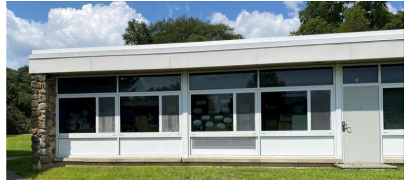
Typical windows at the 1960/64 wing
