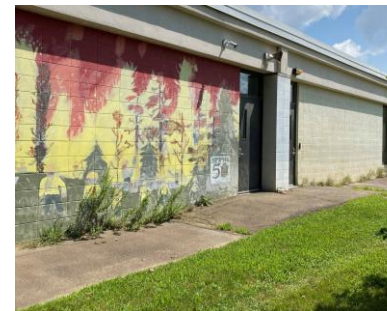
Asphalt paved walk at perimeter of the 1970's central node
