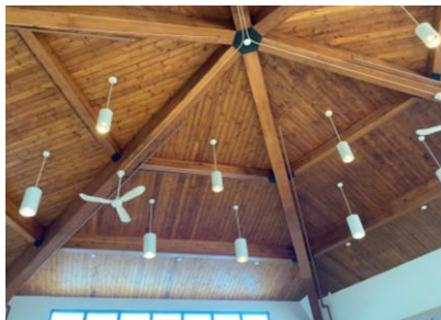
Multi-Purpose Room – Wood plank ceiling
