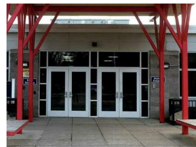
Aluminum and glass doors at North and South entrances.
