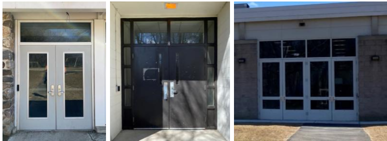
FRP and glass doors Hollow metal doors, 1970 Aluminum and glass doors, 1997
