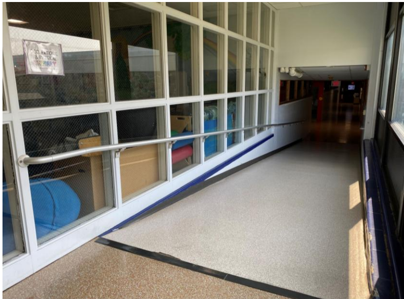
Ramp outside the Commons/North Gymnasium
