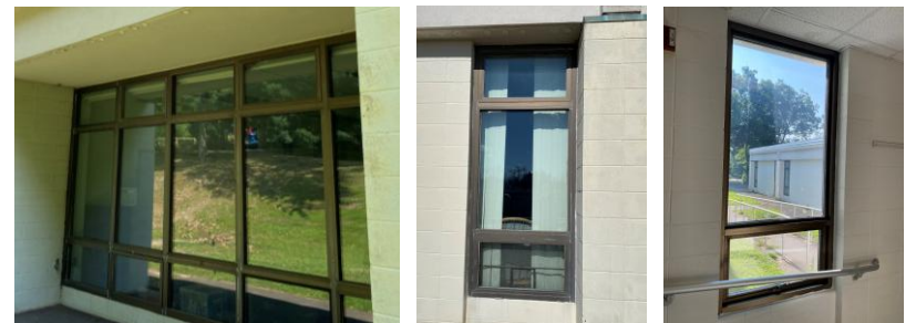
Typical windows at the 1970 addition
