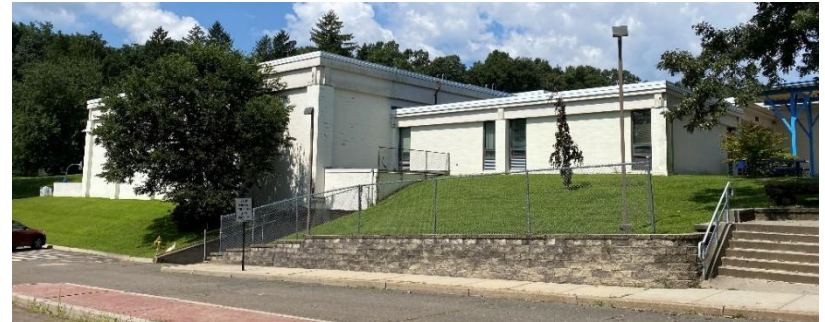
South West elevation 1970 wing. South entrance.
