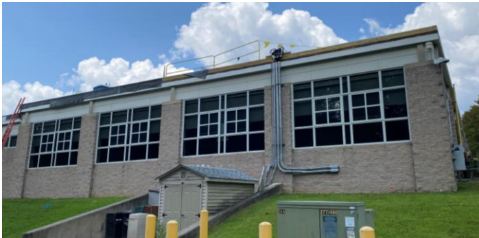
Typical windows at the 1997 addition
