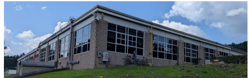
1997. North east façade. Split face CMU and storefront windows.
