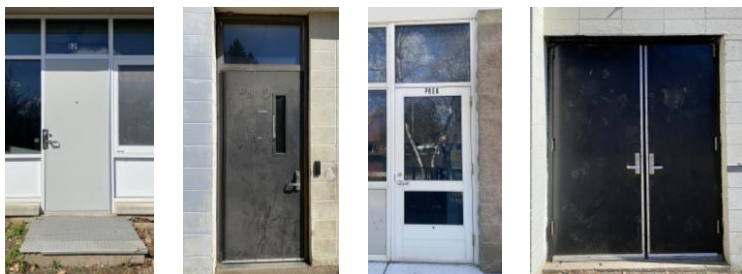
Typical FRP door, 1960/64 Typical metal door with vision lite, 1970s Typical aluminum and glass, 1997 Metal doors at south gym
