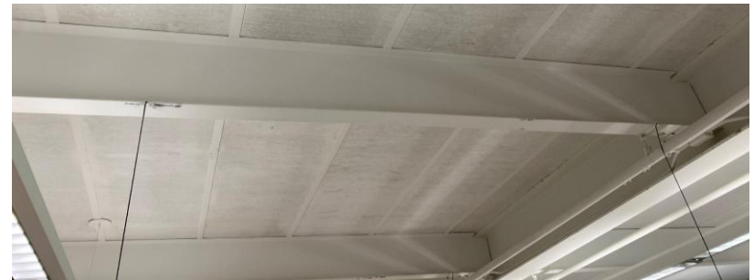
Typical tectum ceiling in a Classroom
