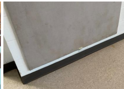
Stained acoustic wall panel
