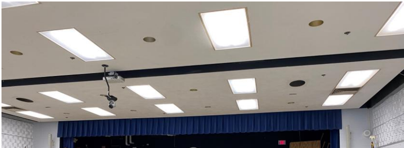
Gypsum board ceiling in the Assembly Space
