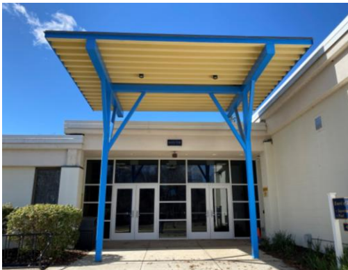
South entrance canopy
