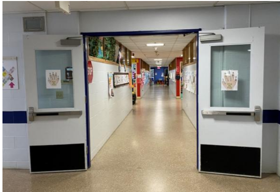
Typical Corridor doors.
