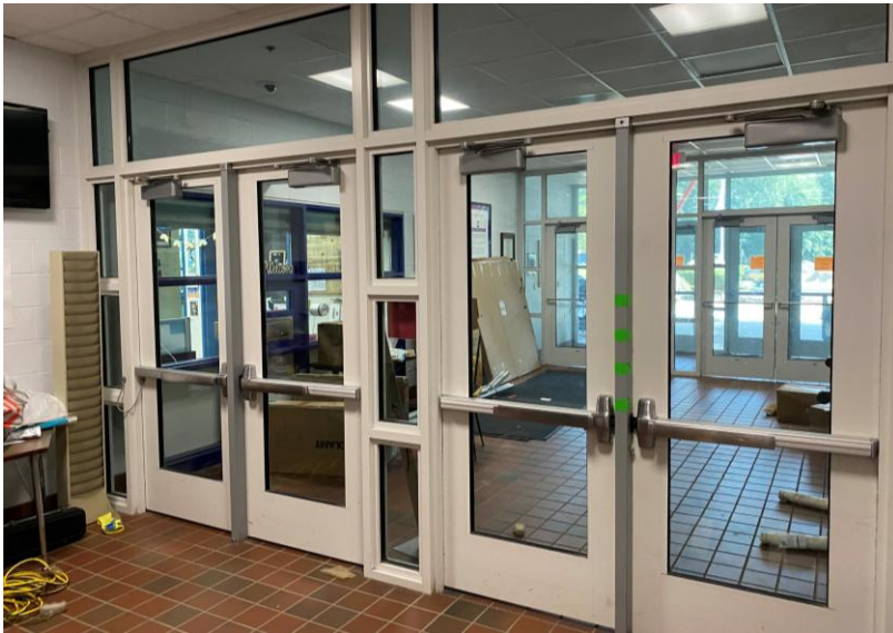
Entry vestibule, North Entrance
