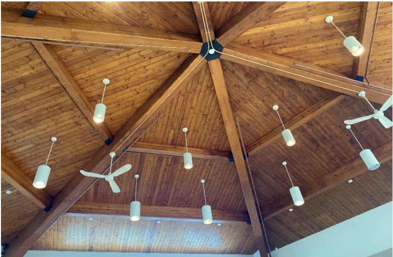
Wood Ceiling in Multi-Purpose Room
