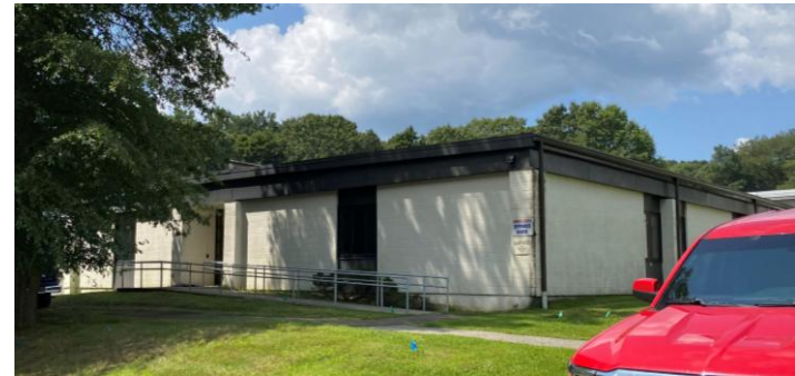
Metal downspouts and gutters at 1994 addition.
