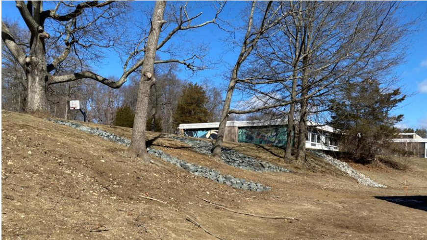
Evidence of regular maintenance: new riprap at grade change
